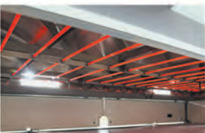
Heating by tube heater
